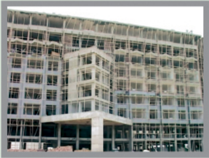
Con-Lub used in superstructure concrete
