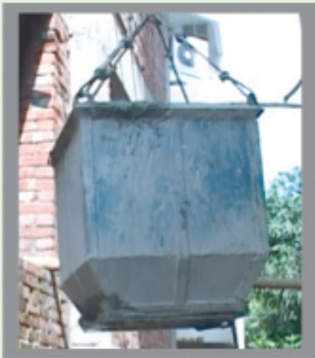
Carrying Con-Lub mixed concrete
