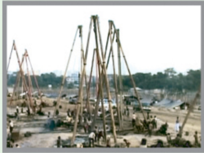
Con-Lub used in pilling concrete
