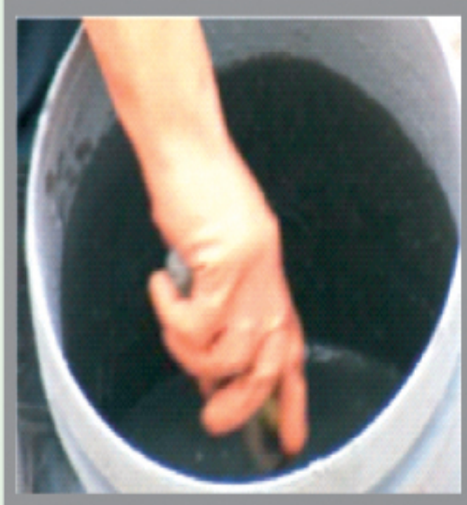
Preparation of cement grout with Foam -Lub (Meta)
