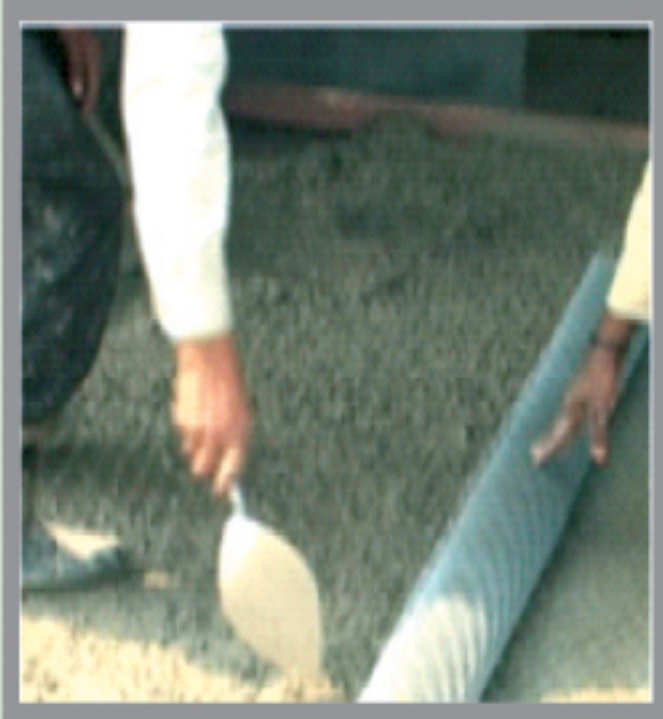
C.C casting with Foam -Lub (Meta) by using wiremesh
