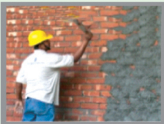
Foam- Lub used in Plaster mortar
