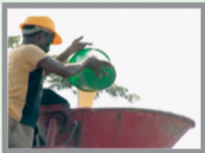
Foam- Lub mixing with concrete
