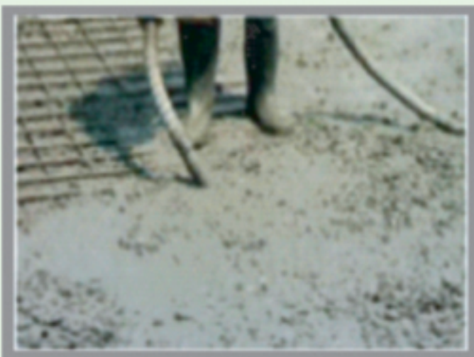
Vibration for better compaction
