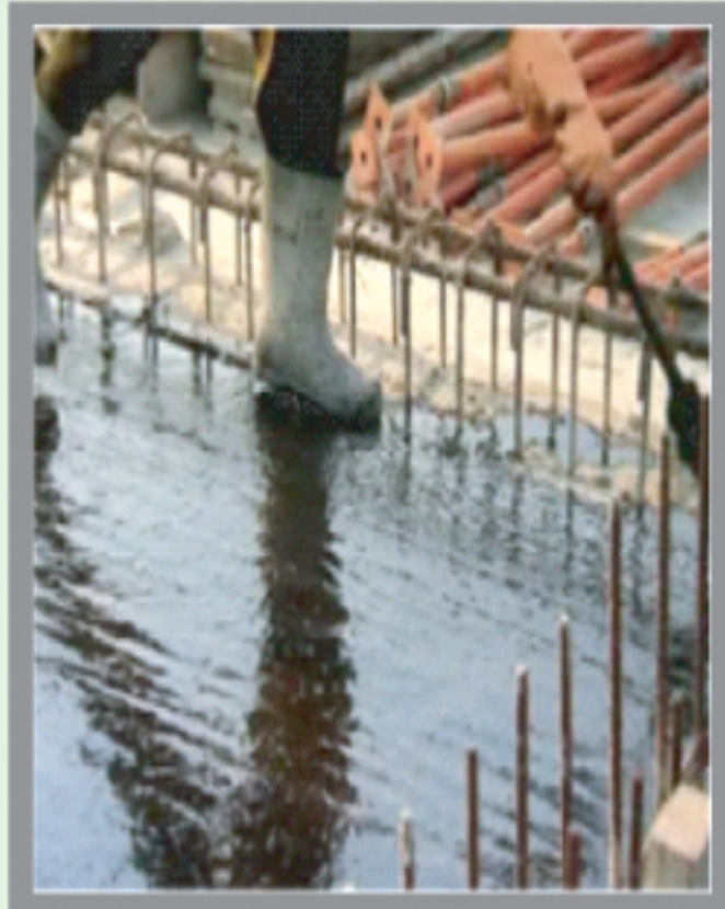
Formation of felt after laying
