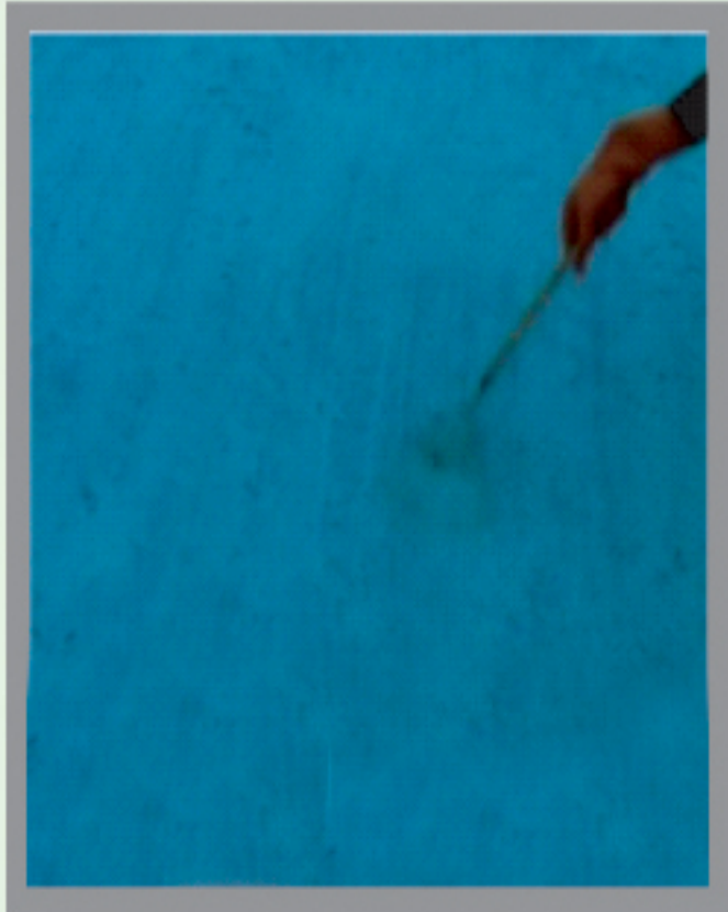
Formation of felt after laying
