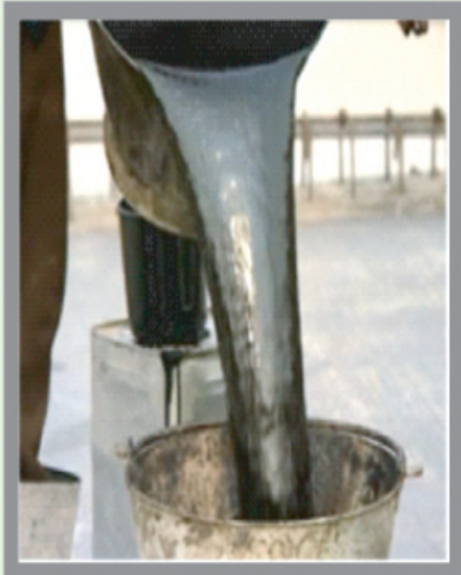
Hydro-Seal, Ef-32 mixing with collar & kerosin
