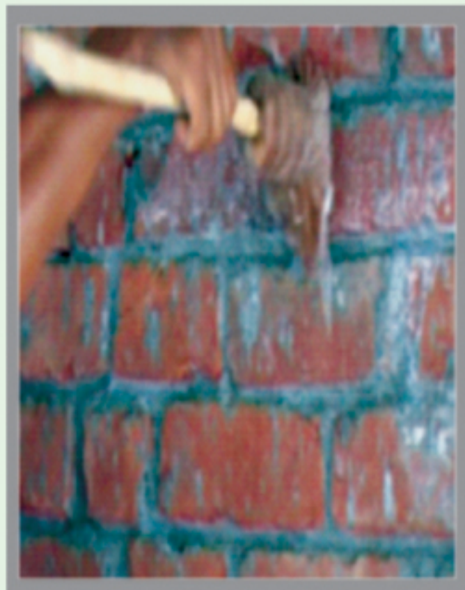
Desalt-S 01 application on bricks surface
