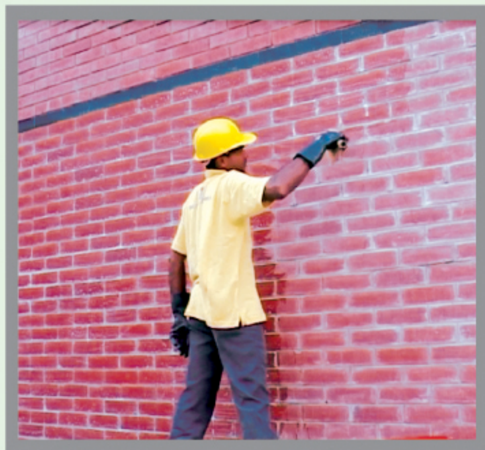
Application of Hydro-Seal, Ef-34 on bricks surface
