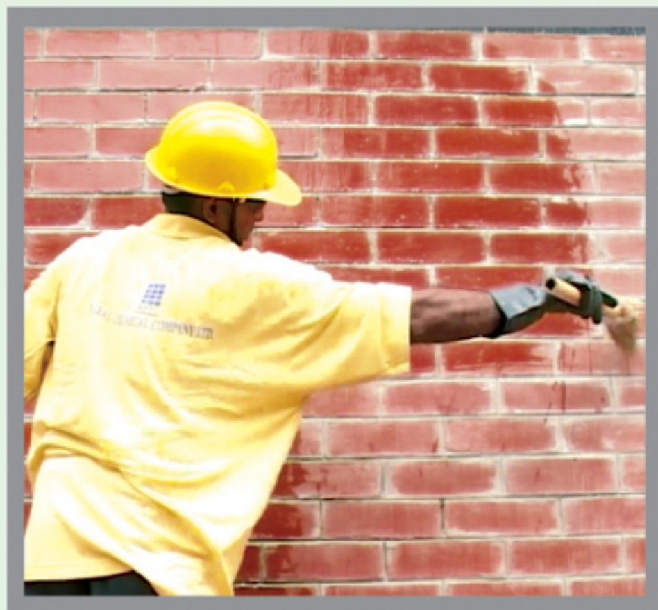
Application Desalt-S01 before using Hydro-Seal, Ef-34
